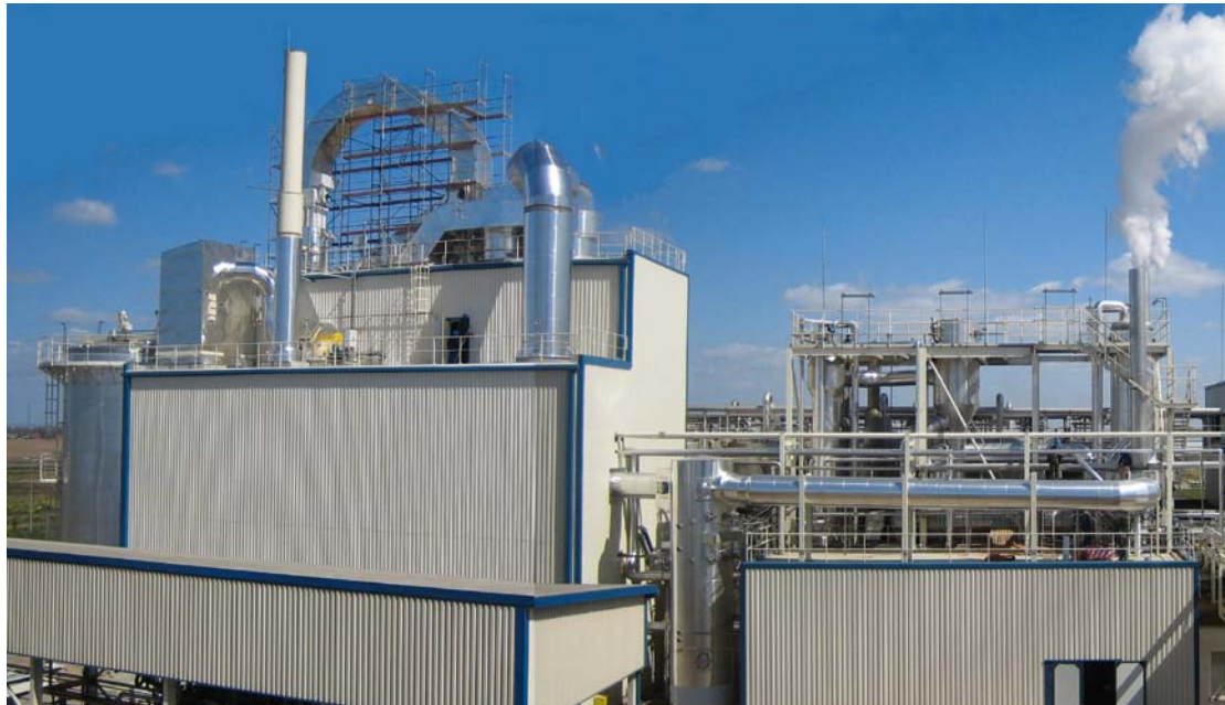
Process line for the treatment of stillage from the production of wheat based alcohol. Energy-optimized combination of evaporator from GEA Wiegand and dryer from GEA Barr-Rosin.
