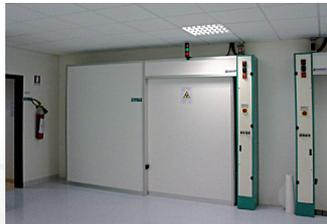
**SPF - Sliding doors with pneumatic movement-fixed threshold**
