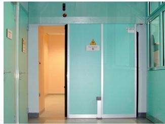
**SFM - Electric shielded door, fixed threshold**
