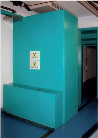
**SPM - Sliding doors with pneumatic movement-mobile threshold**
