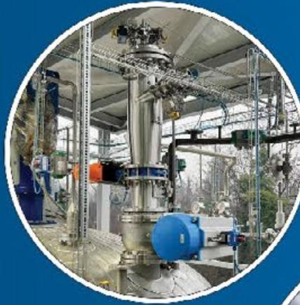
VTS model AGR400 for reactor loading at a height of 10 meters with a capacity of 800 kg/h.
